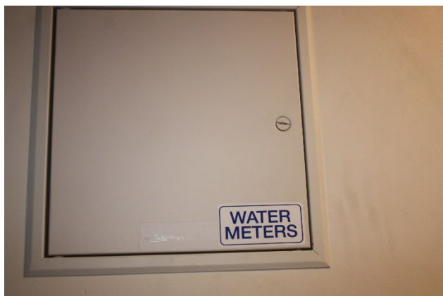
Service access in hallway, for water meter access. Only 2 apartments have a common area where meter access is possible.
