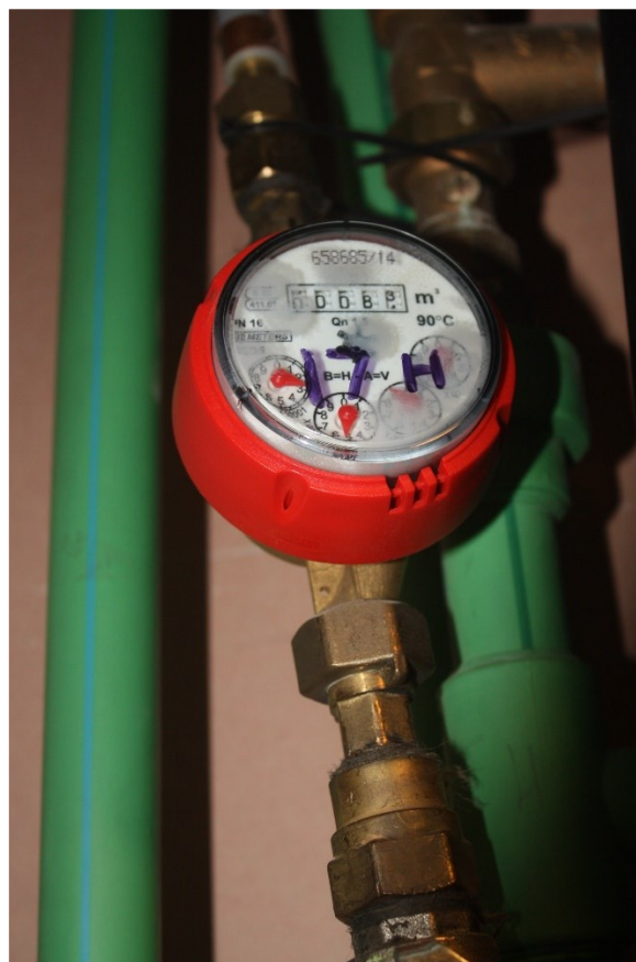
Typical existing hot water meter.
